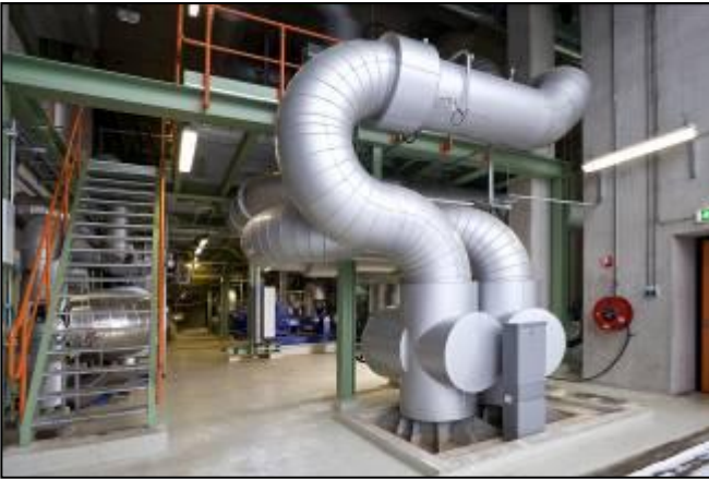
Warmtelevering Essent (80 MW)
