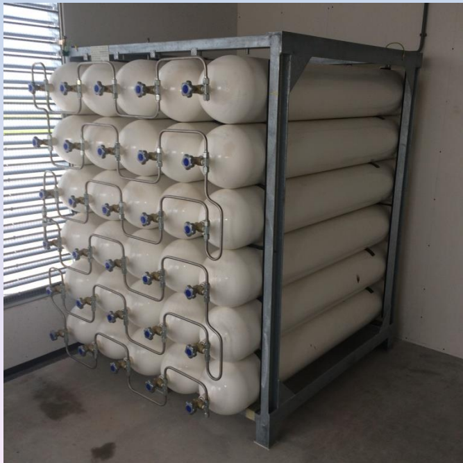
500 Nm 3 @ 200 barg Bottle rack capacity
