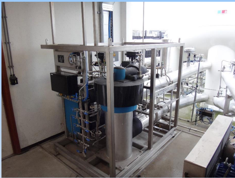
Submerged pump skid
