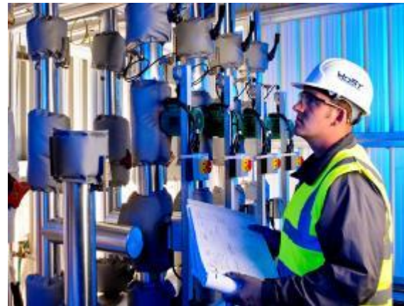
SERVICE & OPERATION 24/7 maintenance team throughout Europe.
